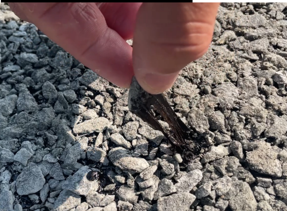
Pictured Above: Pulling a chip out from a 2 day old seal reveals the elastic properties of the CRS-2P emulsion.
